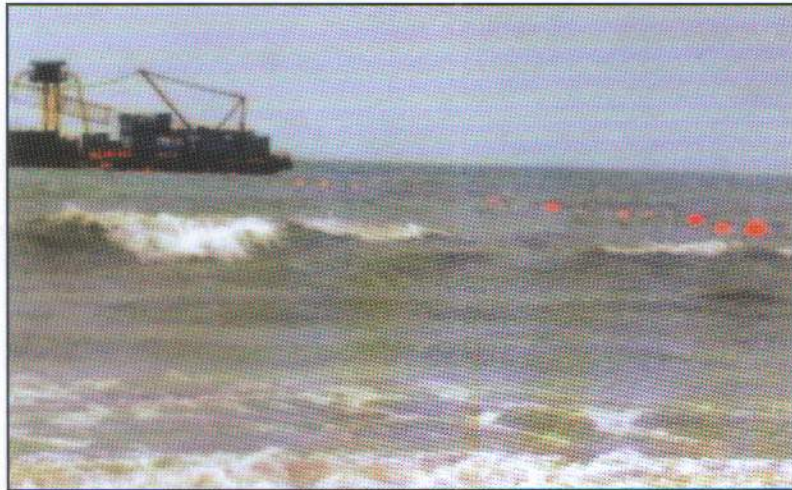
Beach : Cable Landing from barge
