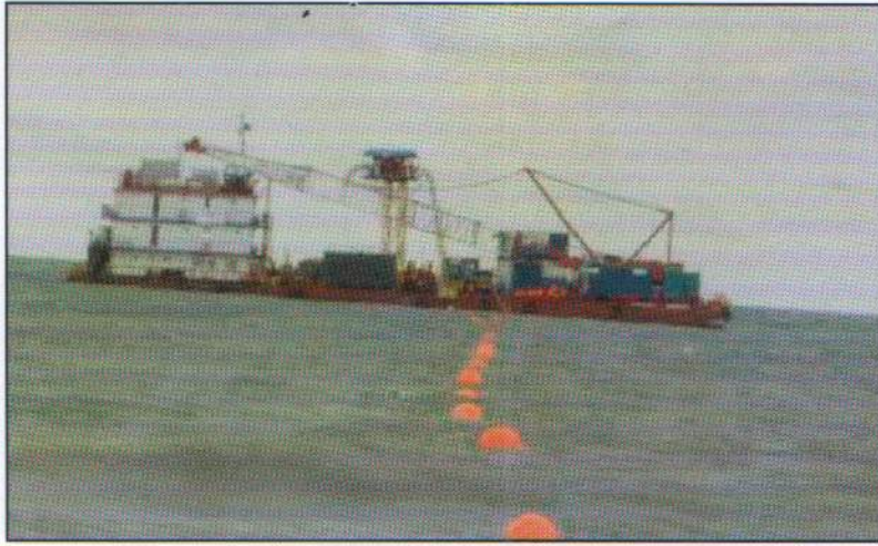
Beach : Cable Landing from barge
