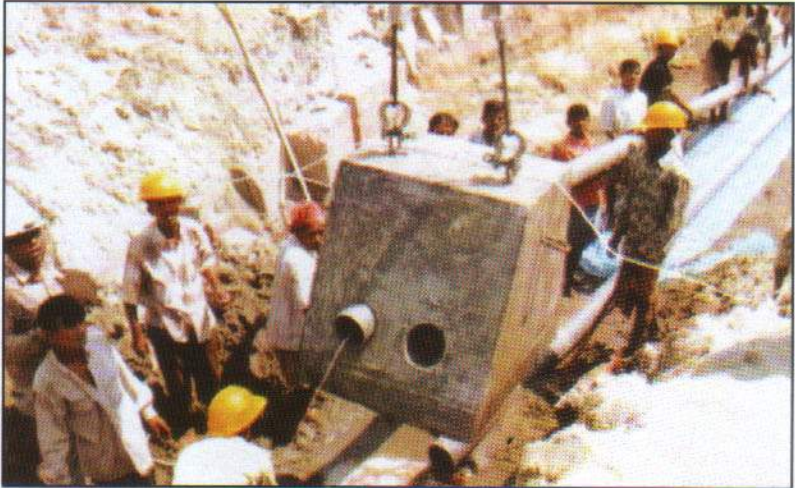
Anchor block placement
